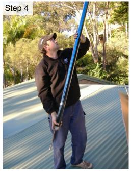
Turn ET up-side-down for 5 seconds, then return to normal position. (This ensures that copper powder returns to bottom of heat pipe.)
