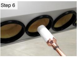
Insert heat pipe into header port, push in full depth. (Heat pipe port is at the TOP of the manifold hole, not centre.)
